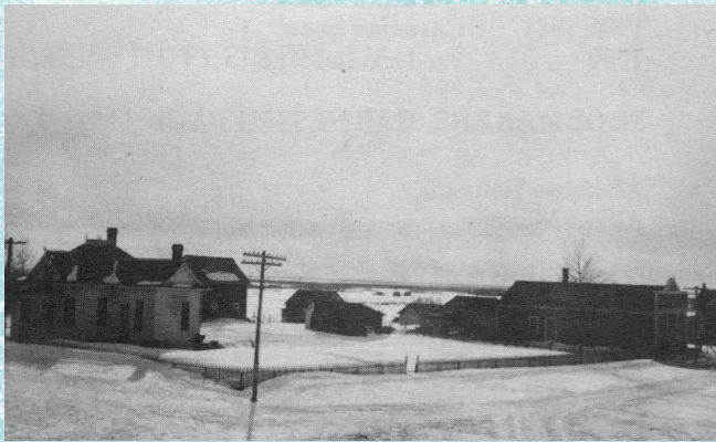
Southwest corner, 50th St. and 50th Ave. (A8986)
